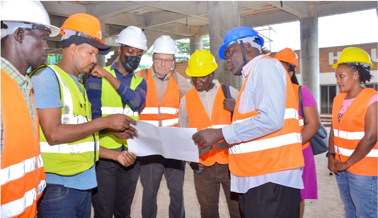
Clerk of works (black mask) explains the construction stages to the team
